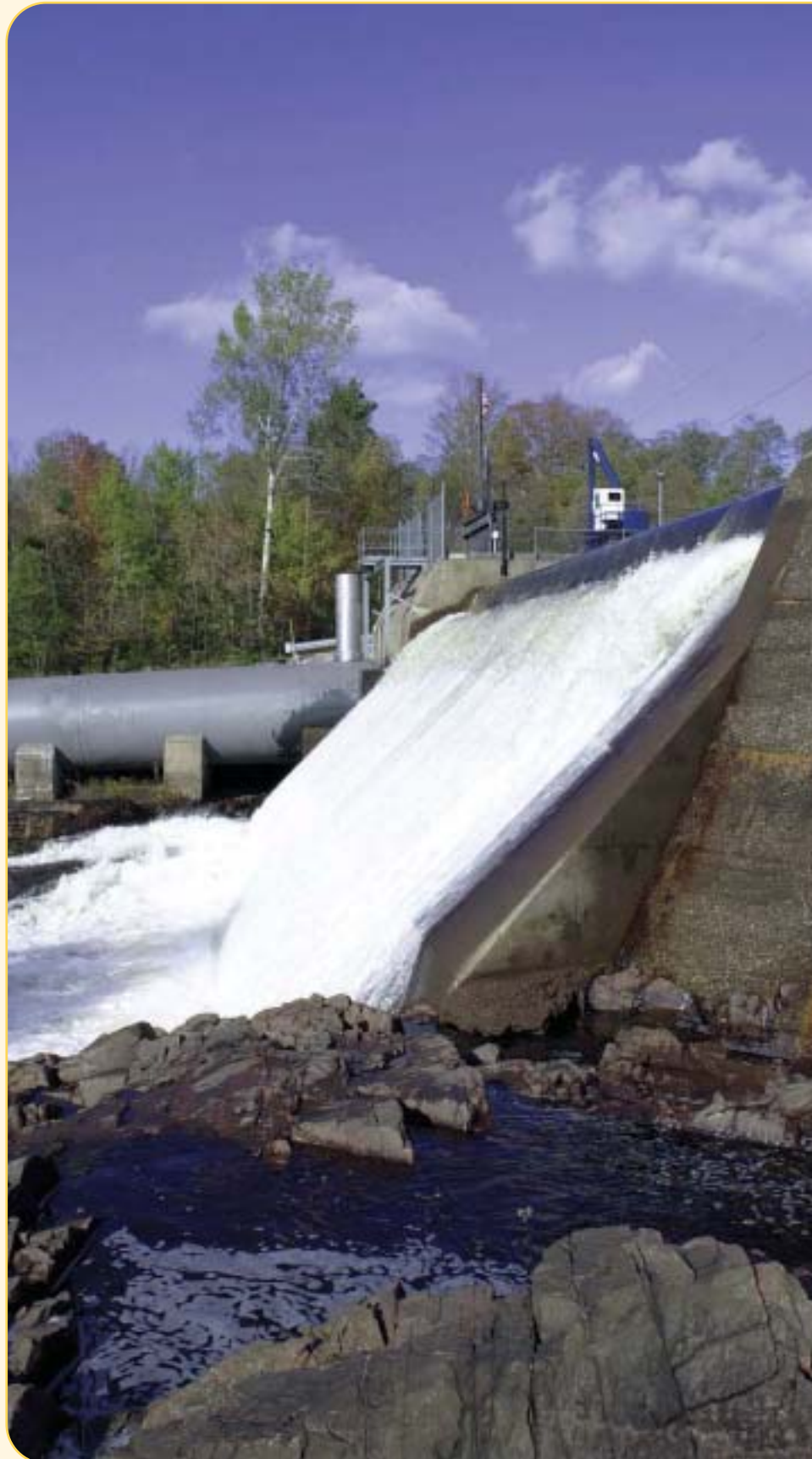
Fortis Companies operate 28 small hydroelectric facilities with 2 more under construction.
